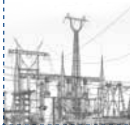
Air Insulated Switchgear
