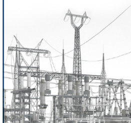
Air Insulated Switchgear
