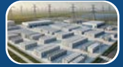
Battery Storage Stations
