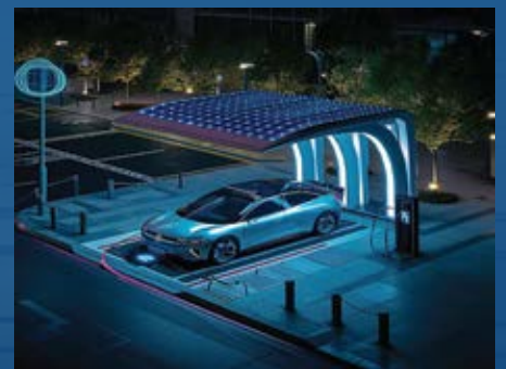
EV Charging Stations
