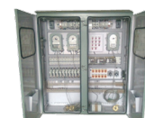
8. Transformer Control Cubicle
